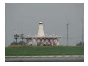
This allows the receiving equipment to determine a magnetic bearing from the station to the aircraft or the line of position (LOP) or RADIAL from the VOR.
